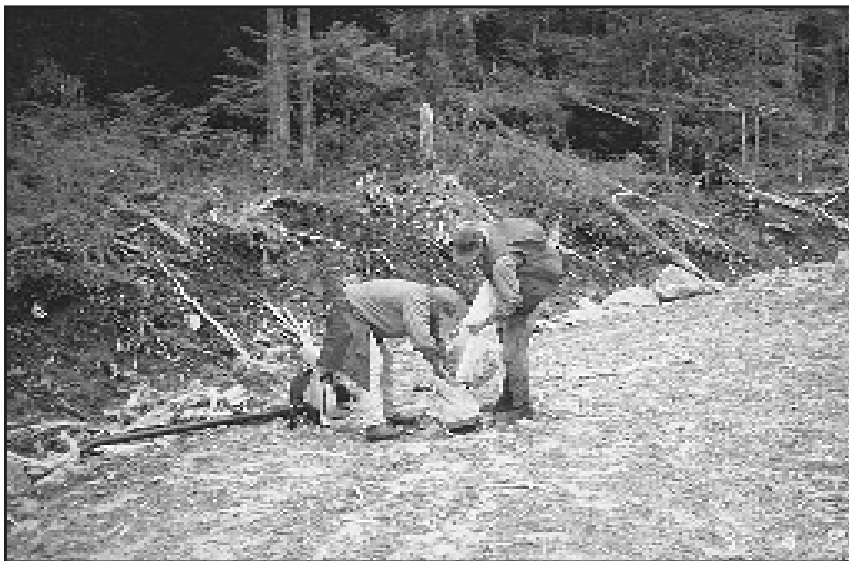
Figure 2. Seeding uphill bank at Goat Harbour Forest Service Road.
