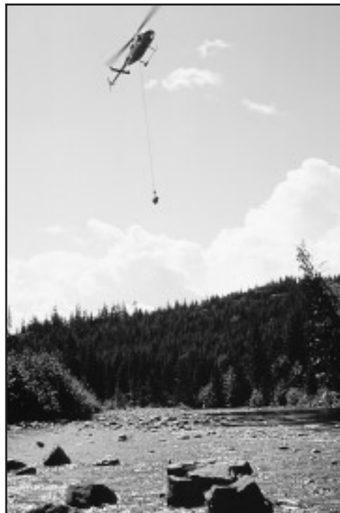
Figure 3. A helicopter carries a boulder in the chain sling and approaches the restoration site. Note the large boulders already placed in the foreground.
