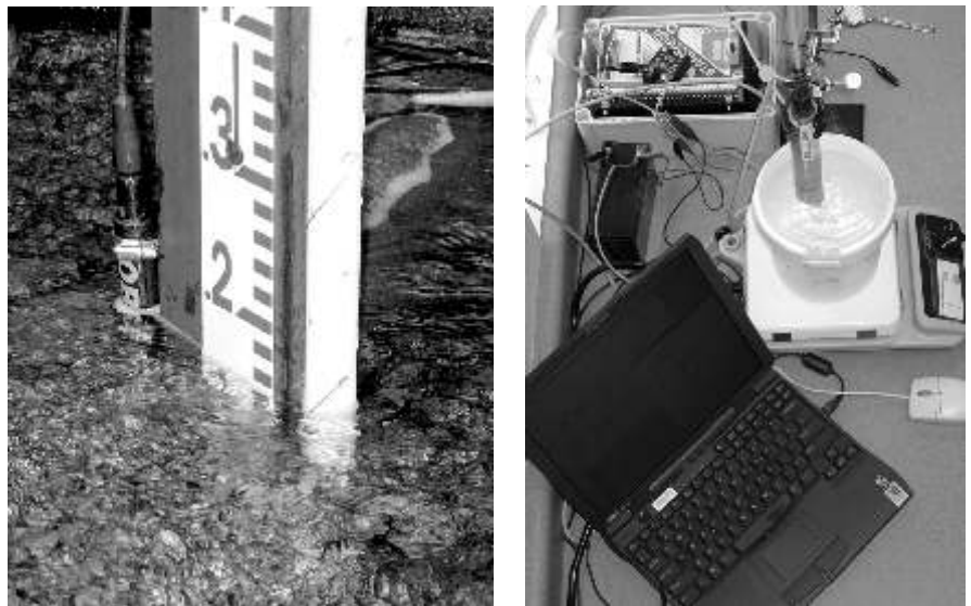
Figure 1. Left: A turbidity sensor installed in a natural stream channel. The OBS-3 probe was originally installed to specifications (D&A Instrument Company 1993), but a peak flow event changed the channel (as shown) and subsequently forced the relocation of this station. Right: An Analite 9500 turbidity probe set up a laboratory. This brand of probe has a smaller "viewing window," which enables it to measure turbidity in a more confined environment.
