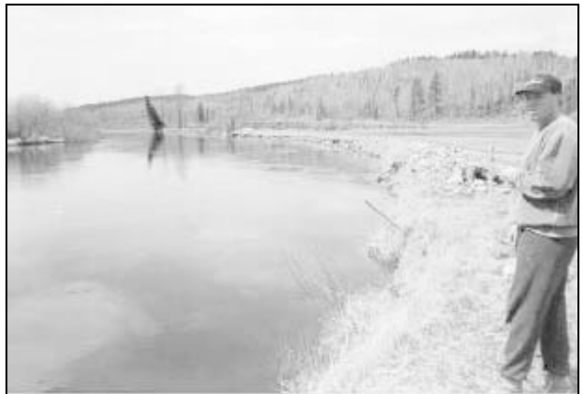
Figure 1. A section of the Horsefly River where debris groins are a bank stabilization option.
