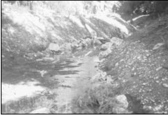
Figure 5. Rock is placed along the toe of the channel to prevent spawning chum from digging into the banks.
