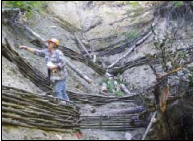
Figure 2. Gully treatment at Cooke Creek FSR 1.7 km. The wattle fences were configured in the form of “arrow heads” to dissipate energy and arrest downcutting.
