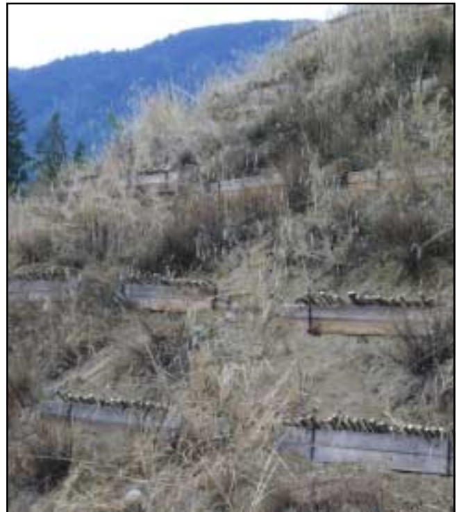
Figure 4. At this site, cedar planks were successfully utilized in modified brush layers.
