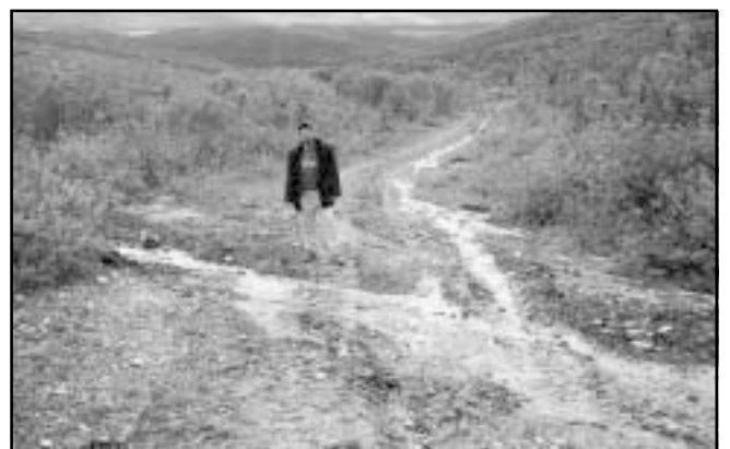
Figure 3. Post-work photo of 4WD Template cross-ditch breached since repairs.
