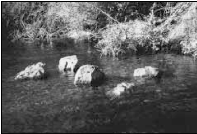
Figure 2. This boulder cluster in the Keogh River is one of the 121 structures constructed as habitat restoration in 1997.
