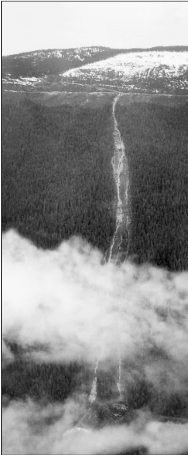
Figure 3. Dramatic example of a debris flow (south mainland coast) that initiated as a minor road fill failure at the junction of two old logging roads.
