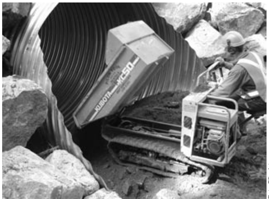
An operator infills a culvert with a power wheelbarrow.
